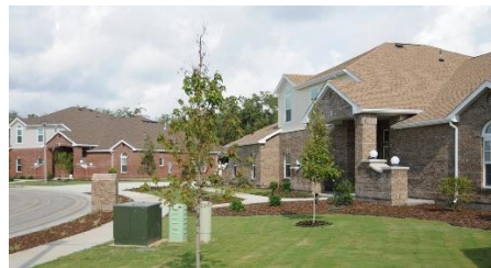
Eleven families from Keesler Air Force Base, Miss., have sued the companies that own and manage base housing there, due to an outbreak of mold that they claim has not been resolved. Some of the families live in the Bay Ridge community, shown here.
