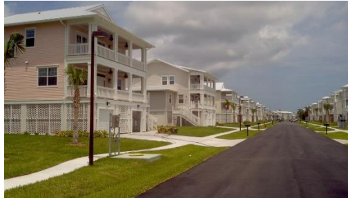
This 111-home family housing development built in 2011 by a private developer at Trumbo Point, an annex of Naval Air Station Key West, is one of many military family housing communities managed by private companies around the country
